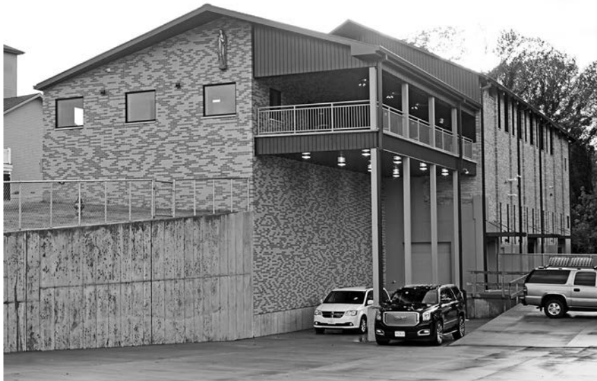
The nearly completed Catholic Charities center in Jefferson City is seen from the parking lot.
